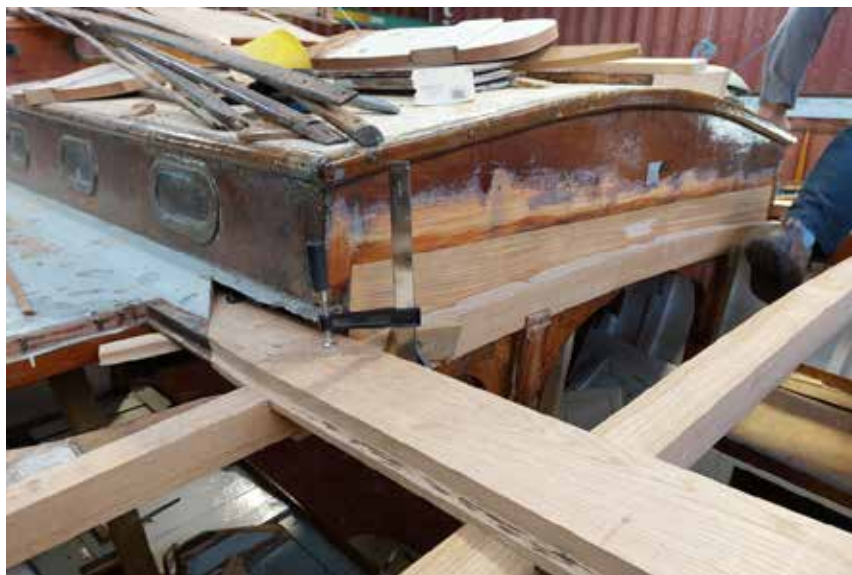
Carlins and deck beams replaced in sawn oak
