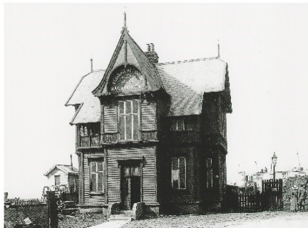
Fig. 6. The Dock Office, Felixstowe, c. 1900, with the heap of coal as described.
